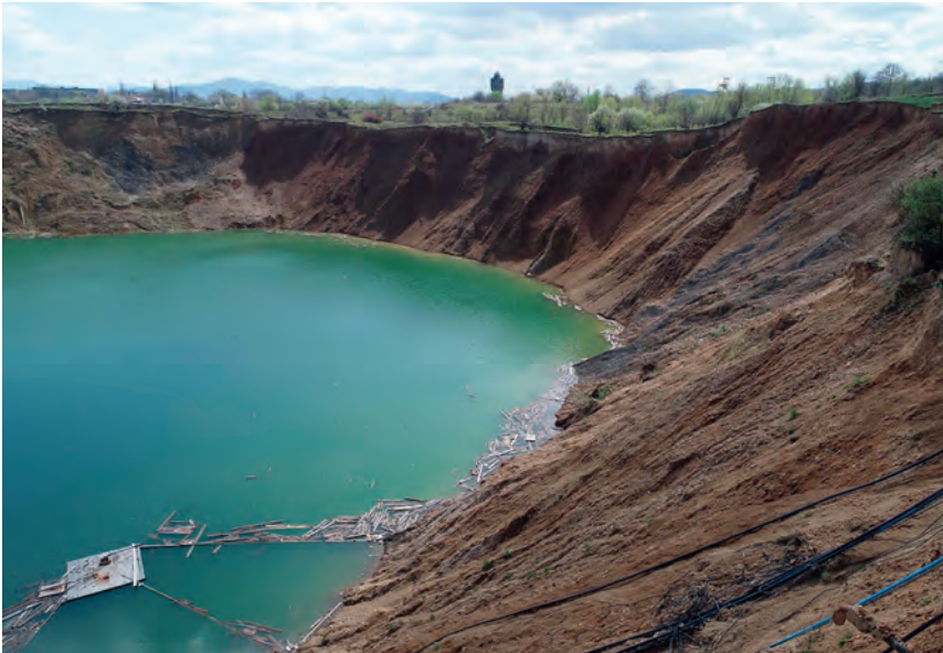
Fig. 10.1.4. Pictures of some sinkholes in the Solotvyno salt mining area (photo by Ivan Prodanets). Flooded mine No. 7 (aerial photography materials as of 2020 was executed using the UAV – Tarot 680PRO Hexacopter)
