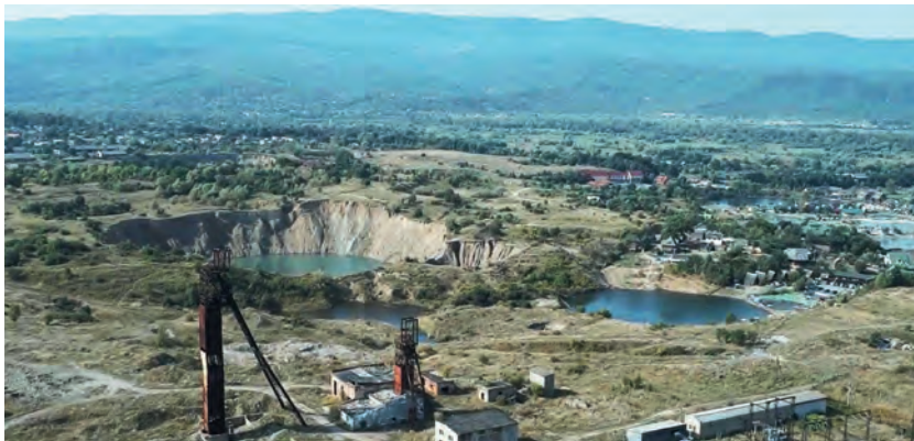
Fig. 5.2.2. Solotvyno salt mine area. Collapse and shear in the mine area. ( https://hromadske.radio/news/2018/07/01/cherez-zatopleni-shahty-u-solotvyni-na-zakarpatti-znovu-mozhe-statysya-obval-foto-video )
