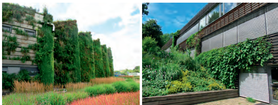
Fig. 9.2. Extensive and intensive green facade in Brno, the Czech Republic (Photo by the author)
