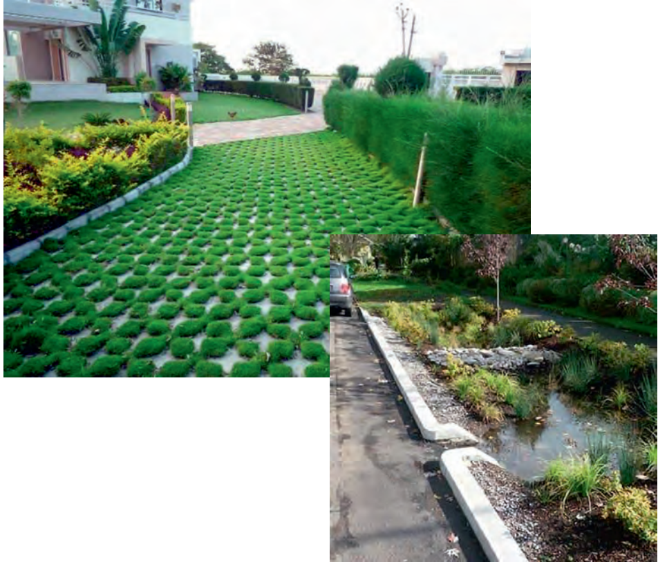
Fig. 9.4. Parking lots with water-permeable surface and a rain ditch (Photo from the Internet)
