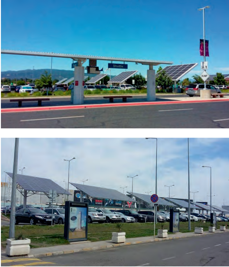
Fig. 9.6. Creating shade and electricity generation at the airports of the city of Medford, the USA and the city of Tbilisi, Georgia (Photo by the author)
