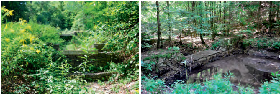
Fig. 9.10. Cascade of barrages in forest ravines, resulting from soil erosion, and in temporary streams of Slovakia (Photo by the author)
